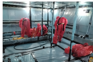
During Bagging Up
